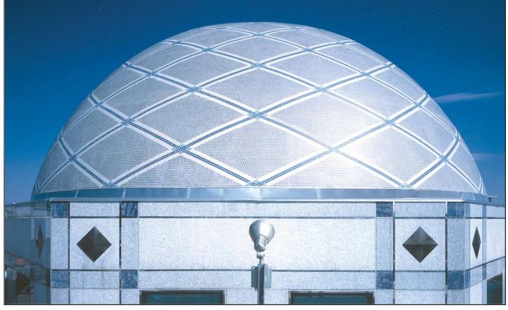
numerous pieces of Mount Airy granite used for the facade were inlaid with 1" wide polished stainless steel bar, and embellished with 1,078 pieces of Azul Bahia granite from Brazil. In addition to sawing a recess in the stone to receive the stainless steel accent bars and drilling holes for the welded studs, a great deal of hand assembly was required. Some of the exterior panels also called for false jointing to create a unique look.
