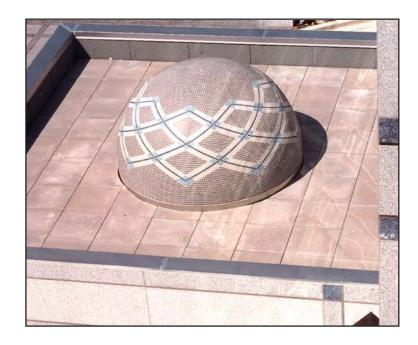
The building's exterior features two domes made of Arabic patterned mosaic tile, which were assembled in the field by craftworkers. Together, the two domes required 2,085 sq.ft. of tile.
