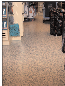
BAC craftworkers from Port Morris Tile & Marble first used MAPEI's Quickpatch for floor leveling. They then placed a combination of 1/8-inch, 3/8-inch and 1/4-inch zinc strips into panels ready for the matrix/binder and broadcasting of aggregate.
