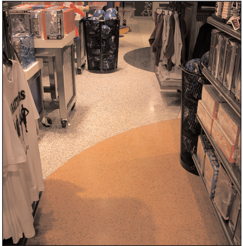
Because of the quick set and grind times of the Terratop system, merchandise was placed in the retail area almost immediately following the installation.
