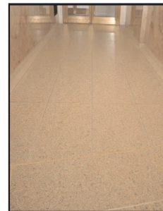
BAC craftworkers from Port Morris Tile & Marble first used MAPEI's Quickpatch for floor leveling. They then placed a combination of 1/8-inch, 3/8-inch and 1/4-inch zinc strips into panels ready for the matrix/binder and broadcasting of aggregate.
