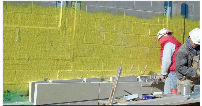
Fluid-applied elastomeric air barrier (yellow material) with transition material on CMU wall—installed by masons.
