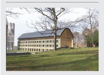
The wall system played a key role in the project's ambition to earn a "Platinum" LEED rating from the U.S. Green Building Council. The AAC units carry an R value around 8, while the rockwool insulation made of 100% recycled material has an R value of 16.8. Exterior stone quarried within 500 miles of the campus, and the "thermally inactive" concrete also helped, as did recycling of construction waste.
