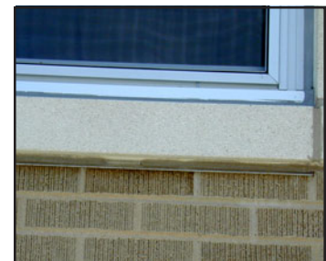
Weep installed under sill
