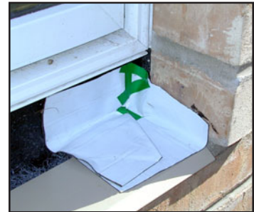
End dams good. Sagging bad. Install through-wall flashing to complete this installation.
