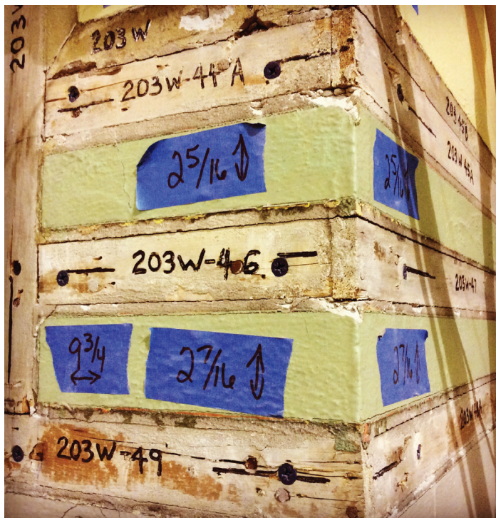
FORMERLY AFFIXED TO THE PLASTER, EACH PIECE OF WOOD TRIM INSIDE UNITY TEMPLE HAS BEEN PAINSTAKINGLY REMOVED, TAGGED AND RESTORED OFF SITE TO BE REINSTALLED UPON COMPLETION OF THE PLASTER RESTORATION.
