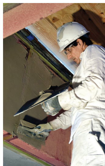
PLASTERER JOHN CZONKA APPLIES A FINISH COAT TO THIS CEILING COFFER IN UNITY TEMPLE.
