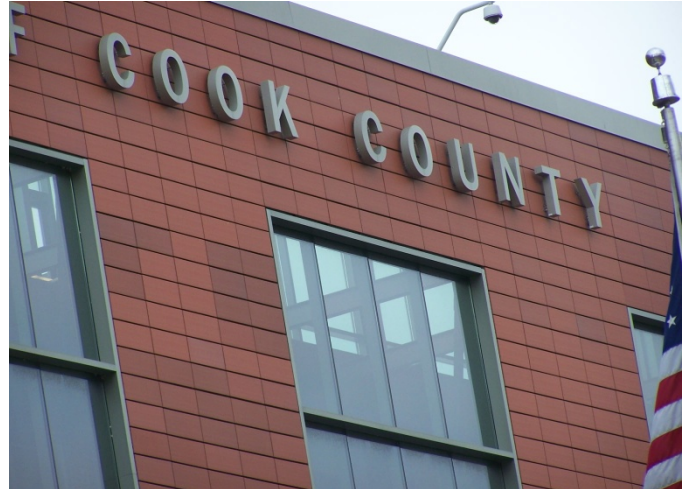
BAC bricklayers installed the rain screen wall on the Cook County Domestic Violence Courthouse in Chicago.
