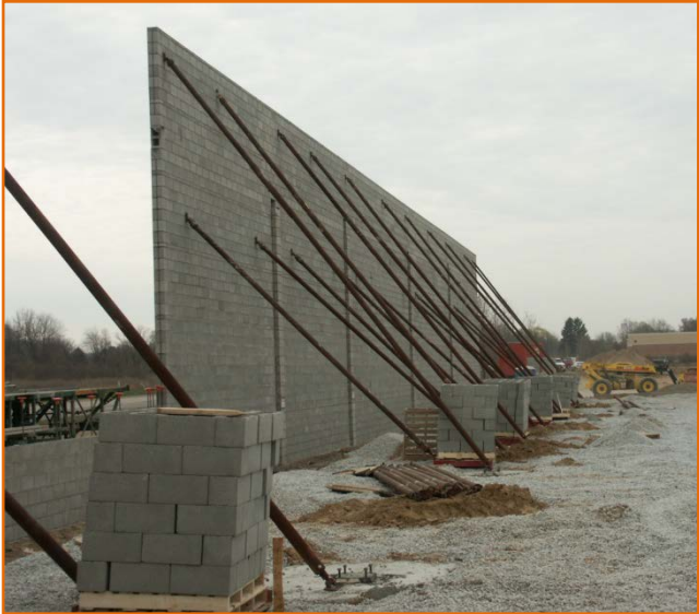
Photograph 1: External pipe braces utilized on a masonry wall under construction with anchorage to block pallet 'skids' and column foundations. (Credit: Davenport Masonry, Holt, MI)
