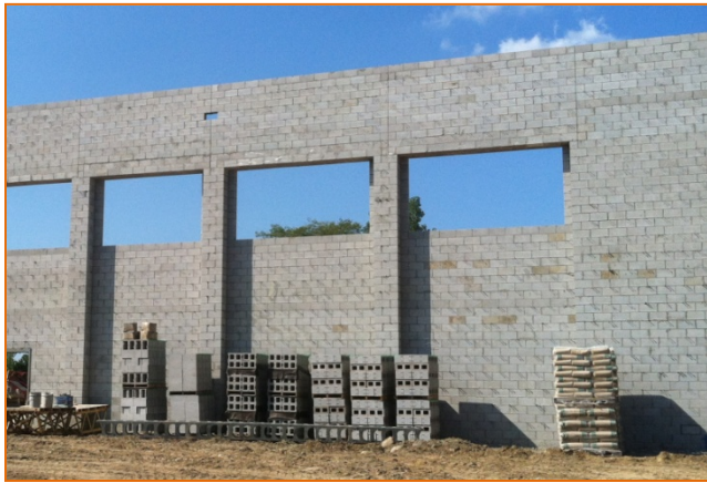
Photograph 2: Masonry walls under construction utilizing Internal Bracing. (Credit: Koch Masonry, Dexter, MI)
