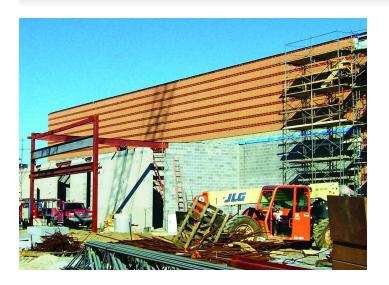
The mason contractor's control of the wall was particularly advantageous with the precast plank. It was set and grouted in one day, while a poured deck would have stopped crews for a week.
