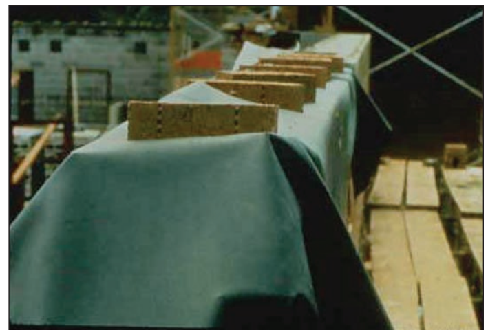
Protect unfinished and finished work.
