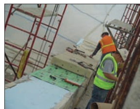
Winter protection for smaller masonry jobs, or smaller areas of large ones, can be a move-as-you-go enclosure.
