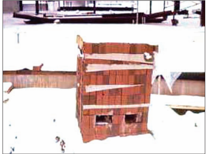
These brick are not properly protected. Protect masonry units from ice and snow and keep dry.
