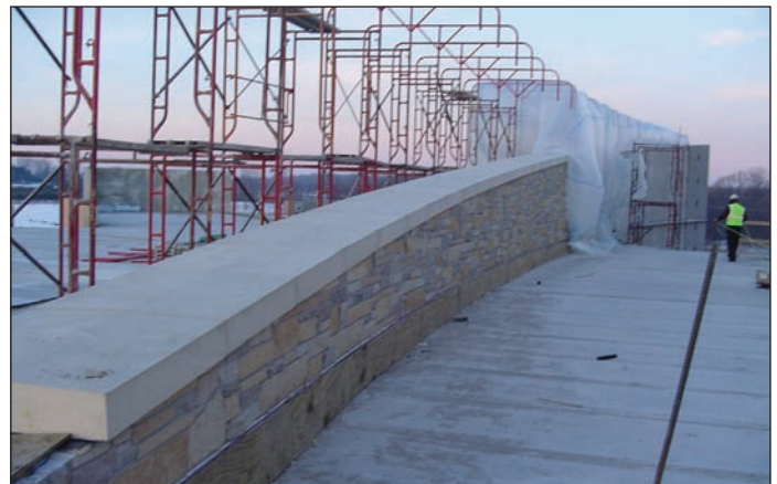
Winter protection for smaller masonry jobs, or smaller areas of large ones, can be a move-as-you-go enclosure.
