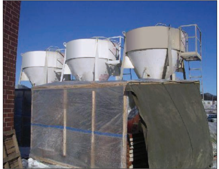
Heated mortar silo enclosure.
