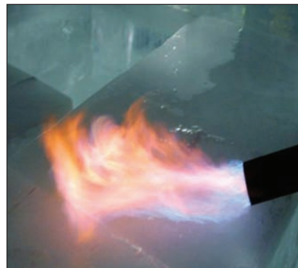
Do not torch units to remove snow and ice. Thermal shock could crack masonry units.
